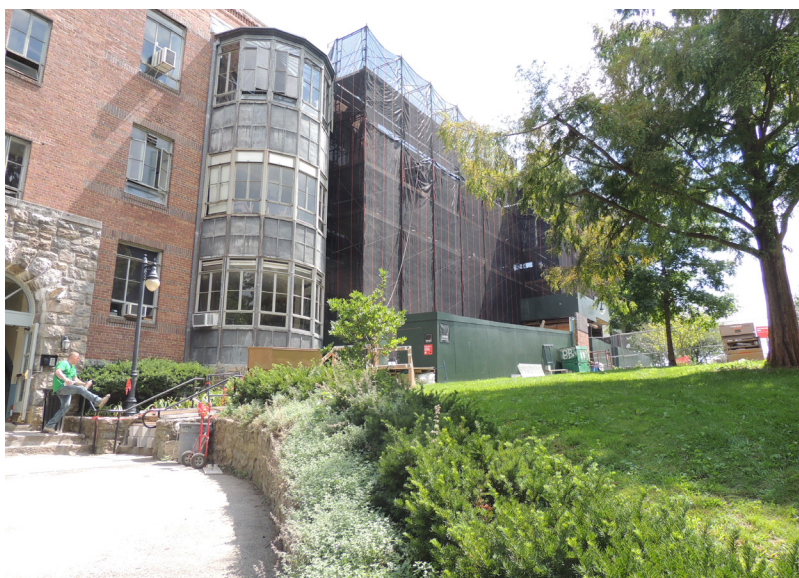
Fieldston Lower School renovations.
